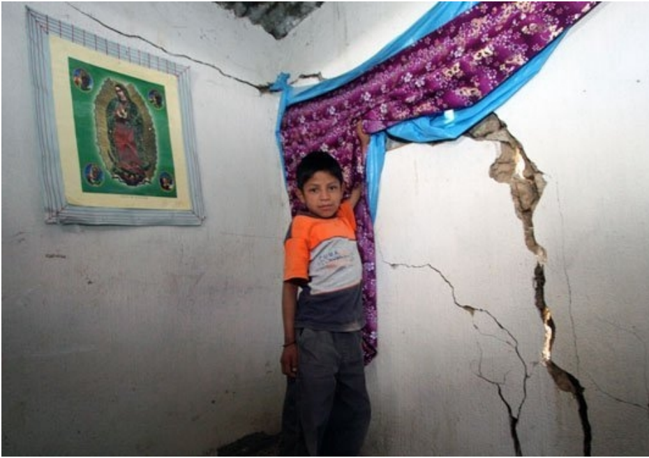
A young boy shows the damage to his home resulting from the mine. Photo used with permission from the Social Justice Committee of Montreal.
